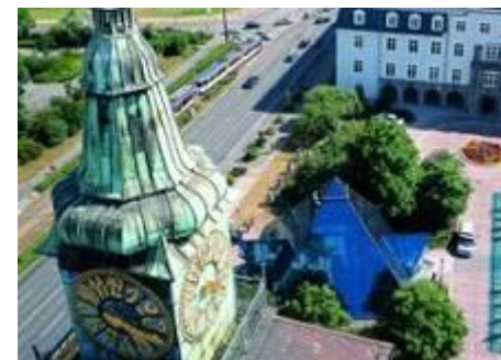
Pützer Tower and Pyramid at Darmstadt headquarters
